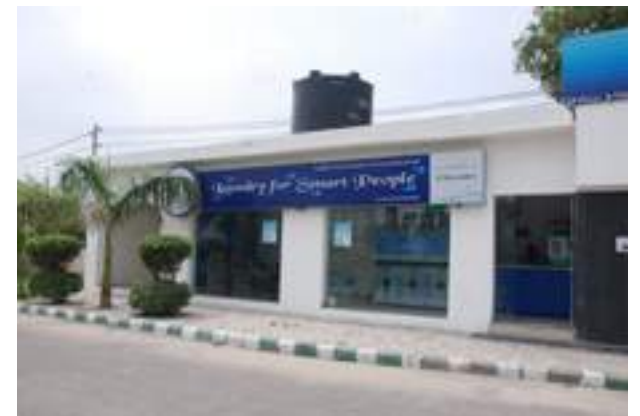
Laundry Facility at SGI
