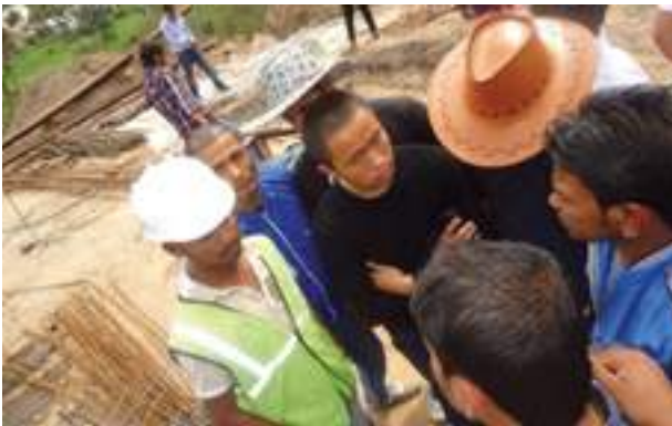
Civil Engineers of SGI at Work on Jammu-Srinagar National Highway
