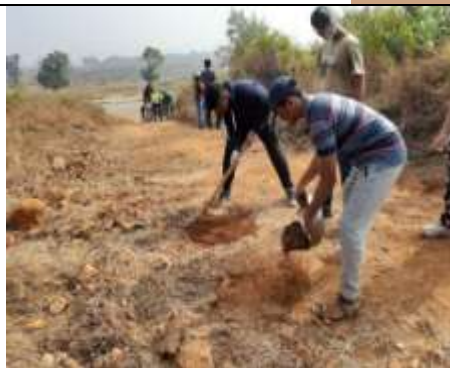
Road leveling project
